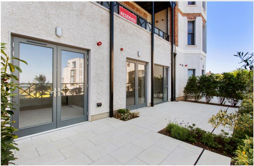
Paving & Walling: Shelbourne Silver Granite Flags (600mm x 400mm x 50mm - Ground) Pembroke Silver Granite Flags (5 size mix x 80mm -Ground) Tara Silver Granite Kerbs (915mm x 125mm x 250mm) Clima-Pave Slane Black Granite Blocks (200m x 100mm x 80mm - Shot Blasted) Clima-Pave Slane Silver Granite Blocks (200mm x 100mm x 60mm & 80mm - Shot Blasted) Tactile Buff Flags (400mm x 400mm x 50mm - Blistered)
